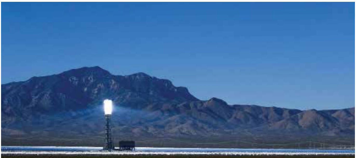
Ivanpah Solar Power Plant, Mojave desert
