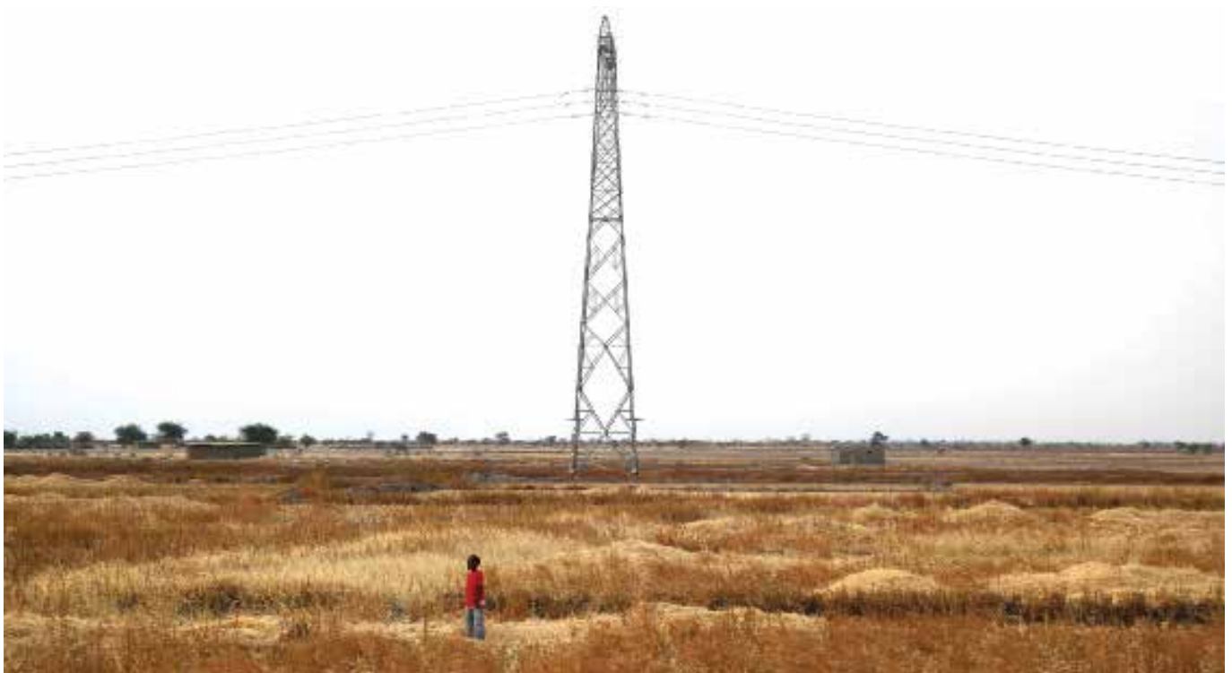
A boy stands under an electricity pylon in rural Tanzania. Over 35 million of Tanzania's 41 million people don't have access to the electricity grid - even many who live close to pylons like this one. © Russell Watkins/DFID
